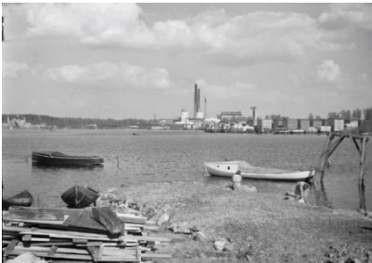
Photograph 1. Time between wars.
