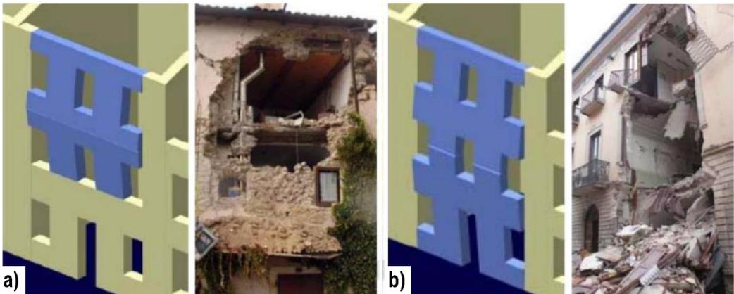
Figure 9. Mechanisms of out-of-plane collapse in presence of an upper kerb: a) partial mechanism; b) global mechanism.
