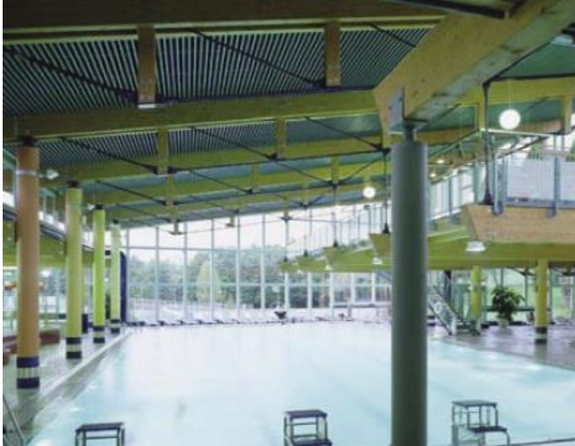
Photo 4: New swimming pool
