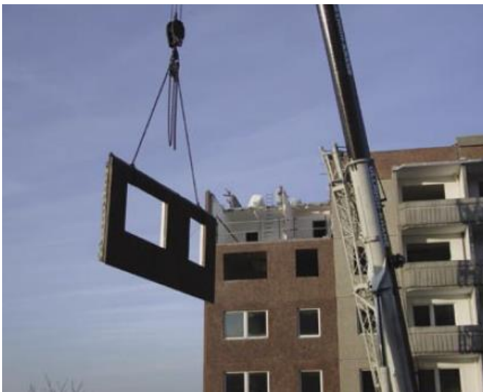
Photo 5: Dismantling of prefabricated houses.
