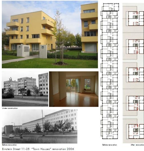
Photo 8: Successful reconstruction of apartments.
