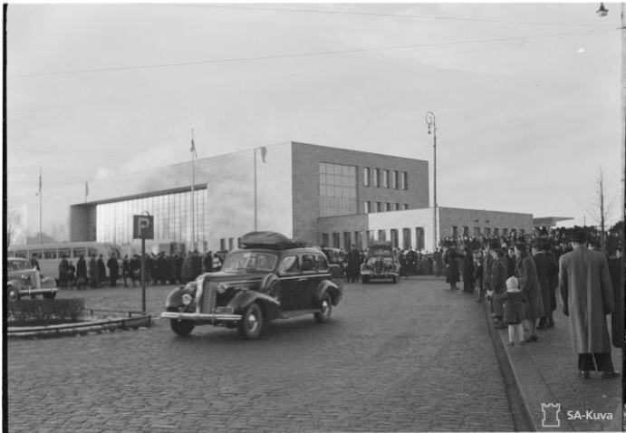
Photograph 1. Turku railway station.
